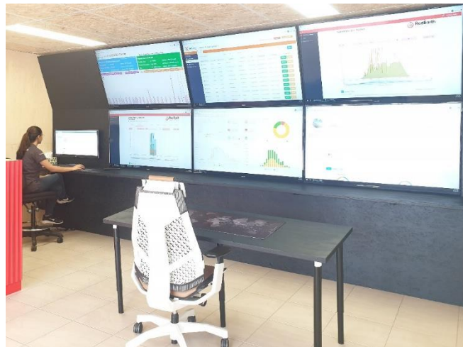
RedEarth's Monitoring and Customer Community Monitoring Visit us in Brisbane
